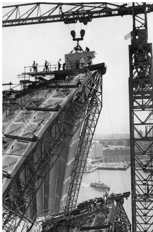
The Sydney Opera House under construction in April 1966. SMH
